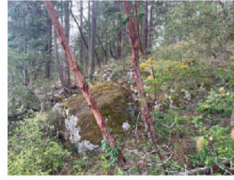
11 As per Golder (1983): "Slope treatment is needed." GES concurs with this recommendation. More broken rocks, indicative of previous rock sliding.
