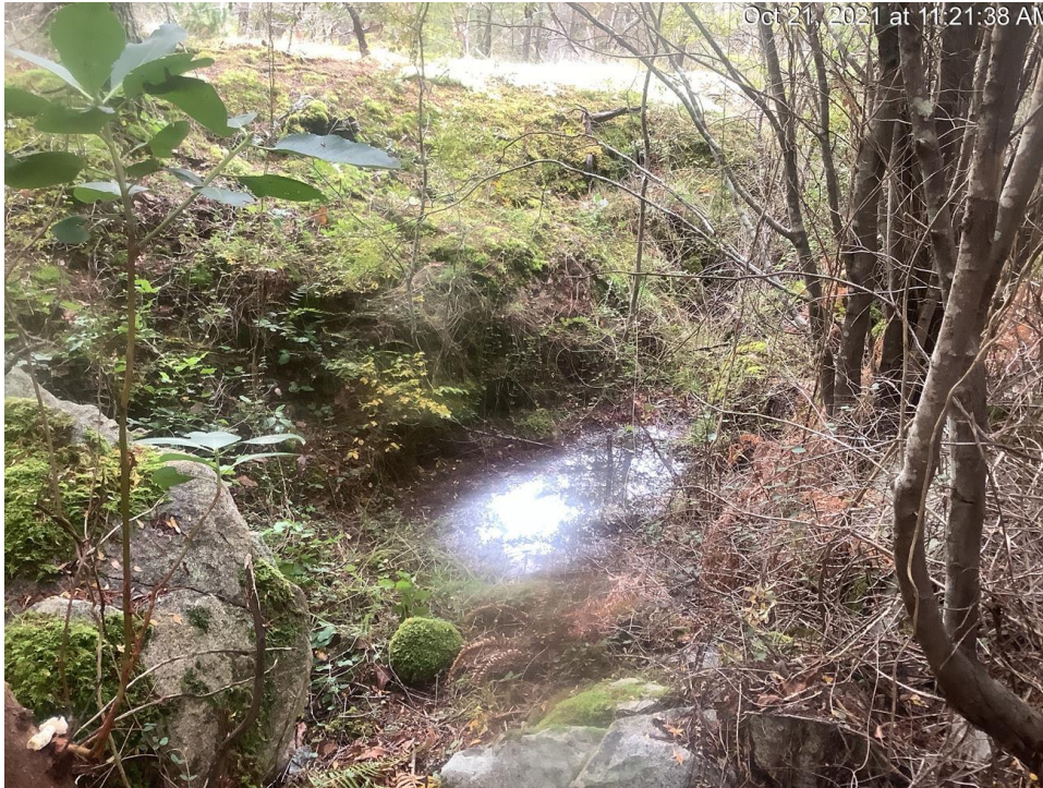
Photo 15. Water pooled in ground depression from rainwater runoff on Truman Road near the western property entrance
