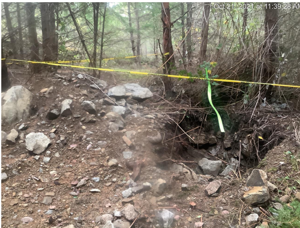
Photo 16. Rectangular excavation within flagged area
